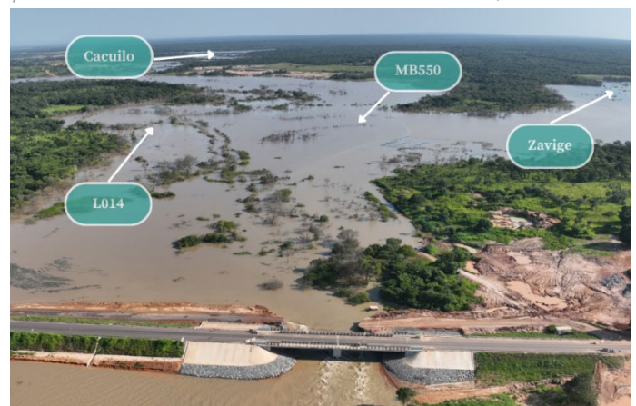
Severe flooding at Lulo; photo taken in mid-April 2024
