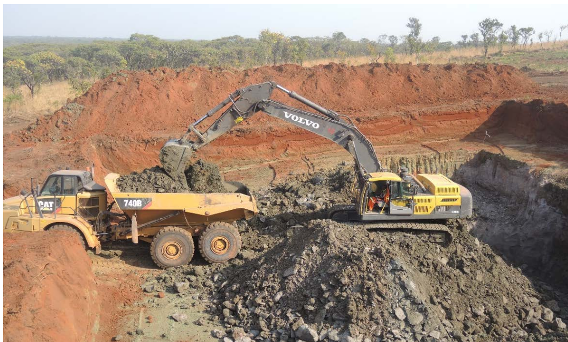
Kimberlite excavation activities at Lulo kimberlite L071
