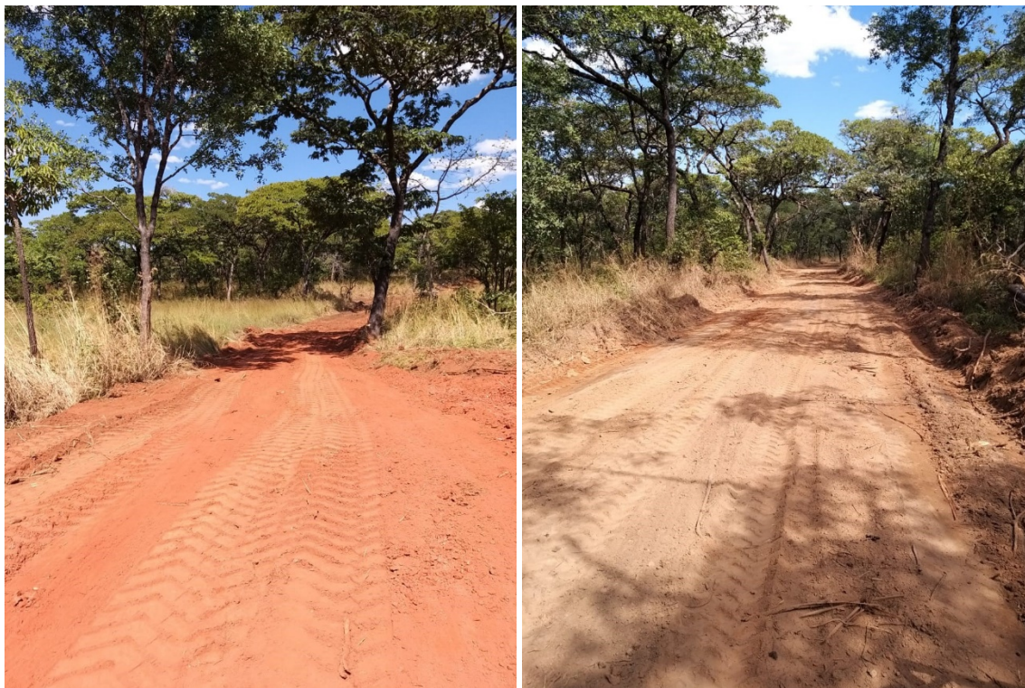
Figure 3: Roads constructed to access L071 in the Canguige catchment
