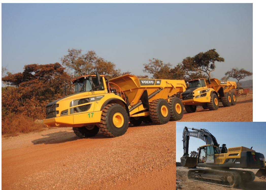
Figure 4: New earthmoving fleet arriving on site at Lulo
