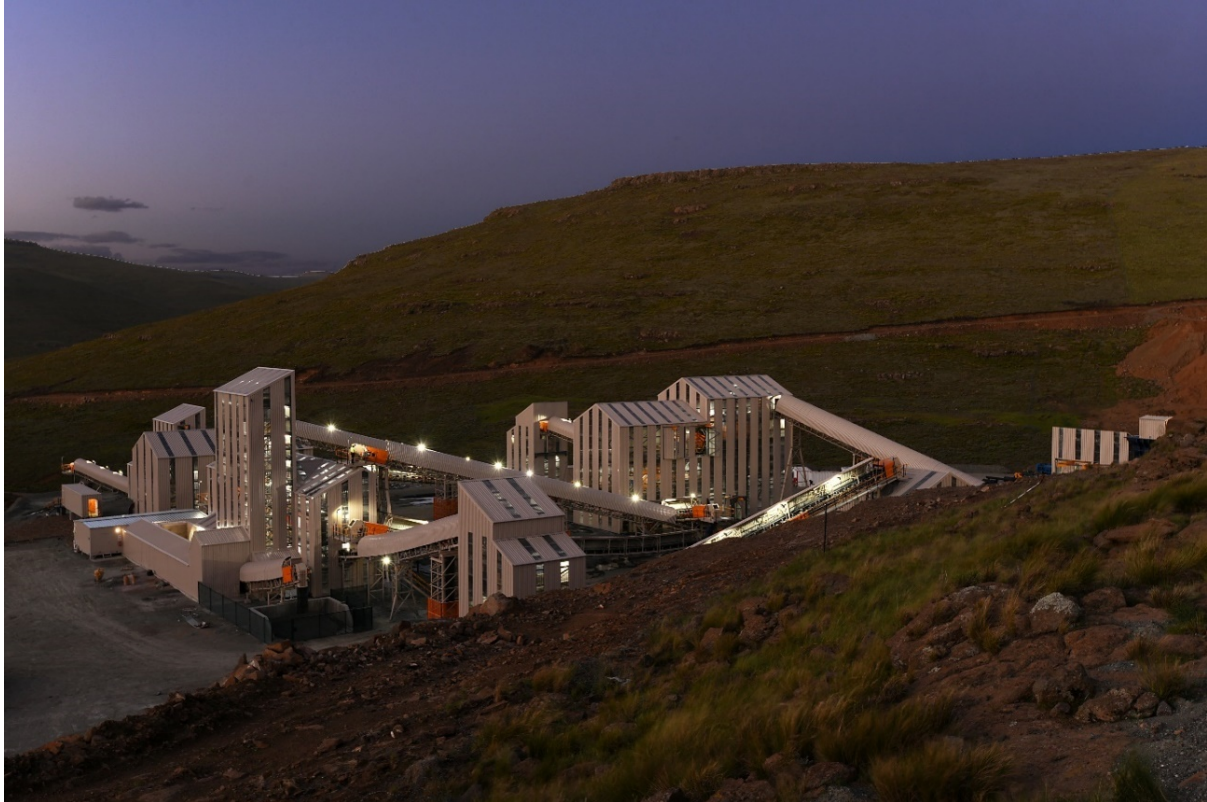
The 1.1Mtpa Mothae treatment plant, which delivered an exceptional performance in its first full quarter of production
