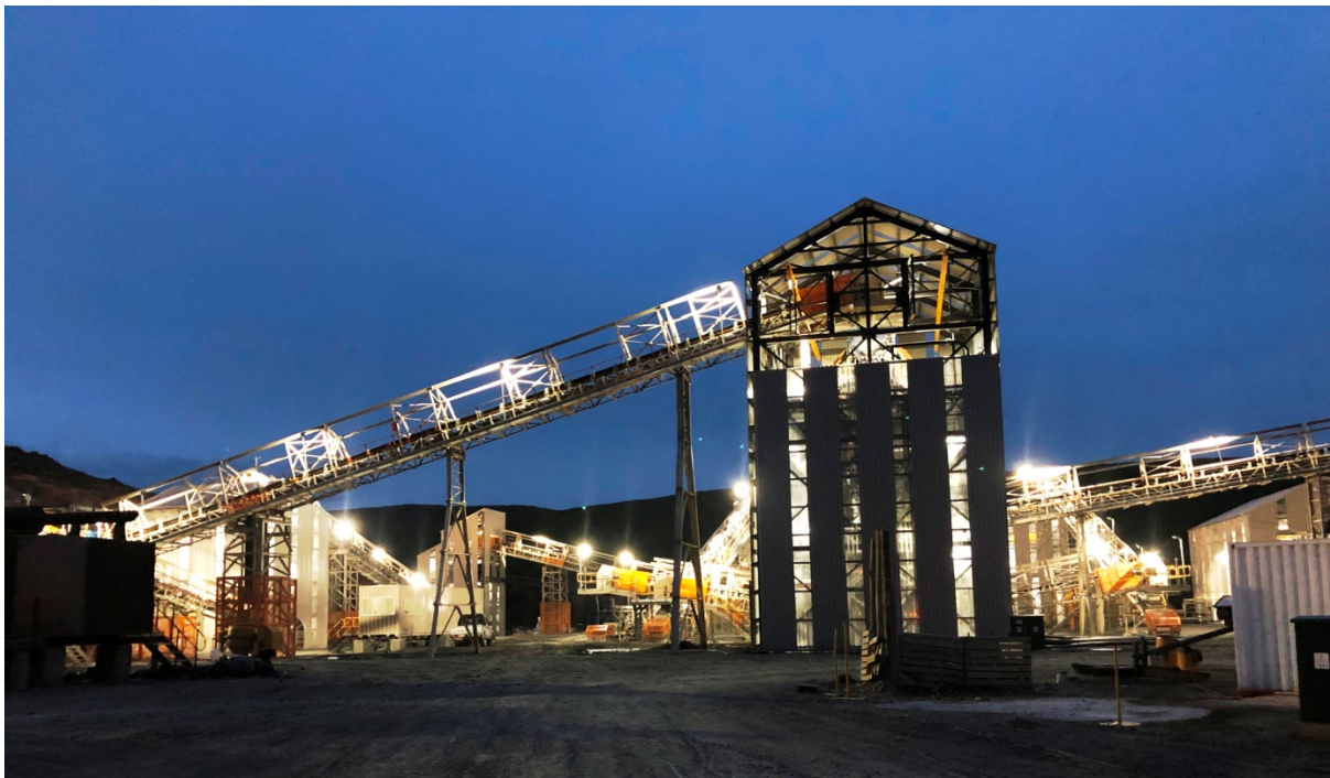
The new 1.1Mtpa Mothae diamond treatment plant completed and commissioned during the Quarter
