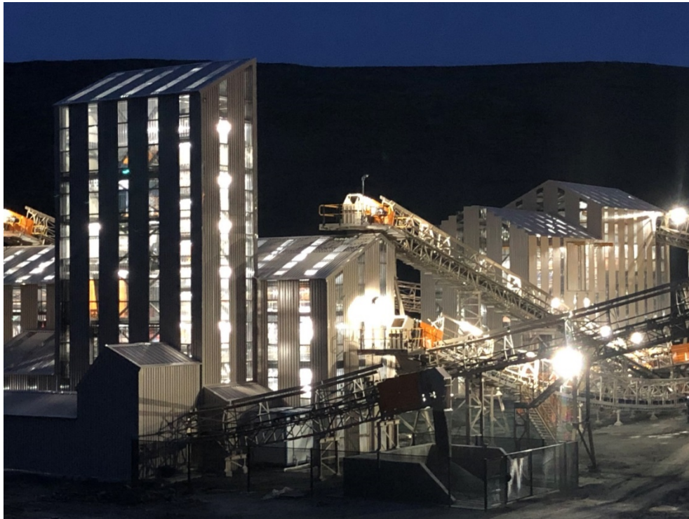
The 1.1Mtpa Mothae treatment plant, which was completed and commissioned during the Quarter
