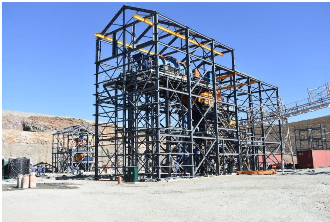
Scrubbing and screening module under construction at Mothae
