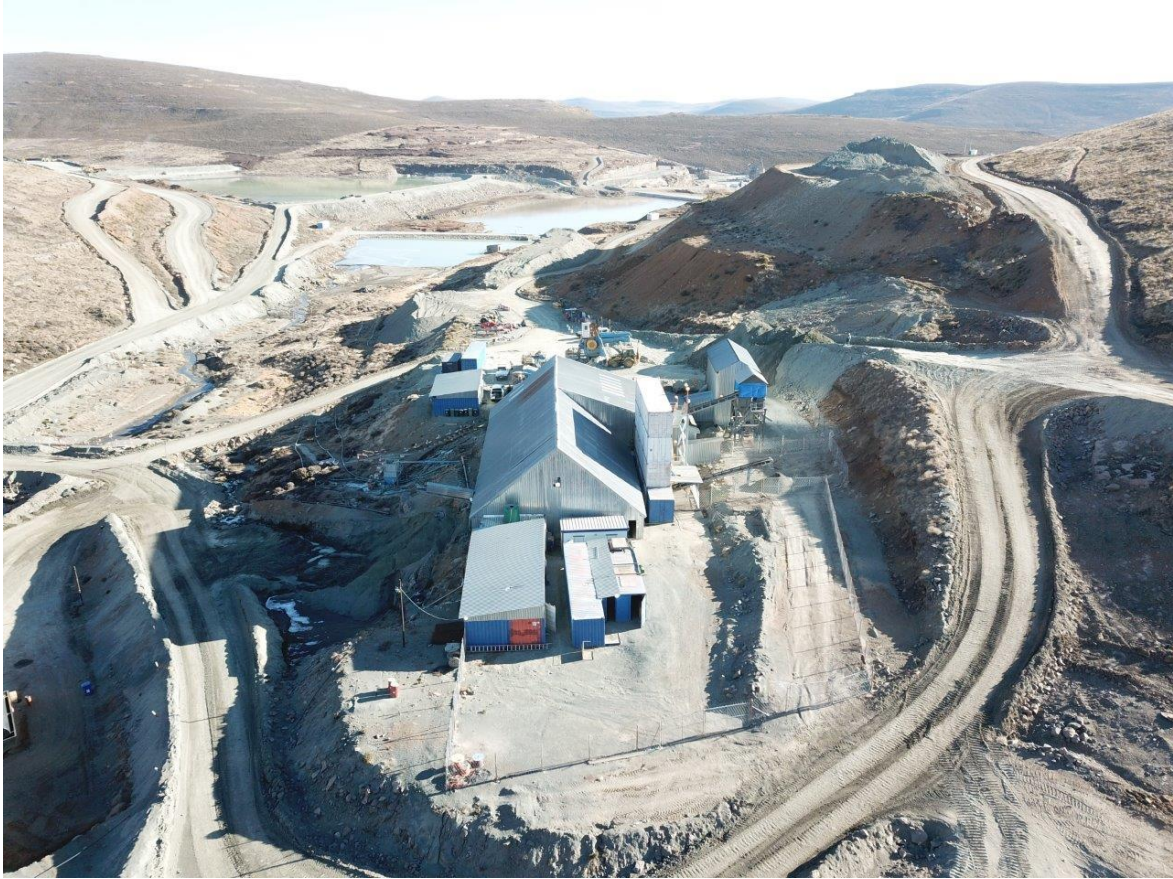
The refurbished bulk sampling plant complex which is testing material from the Neck, South-East and North zones of the Mothae kimberlite pipe
