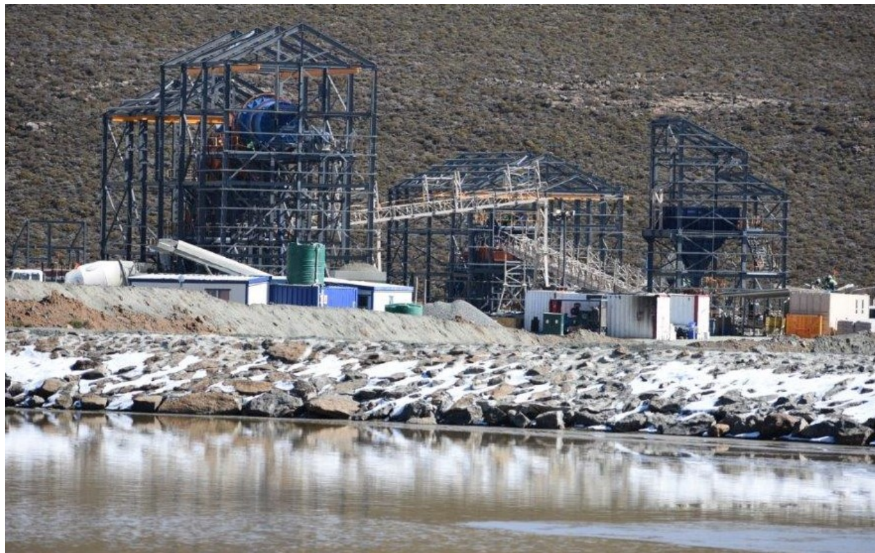
Figure 6: New 150 tph diamond plant, including an XRT large-diamond recovery circuit, under construction at Mothae for H2 2018 commissioning
