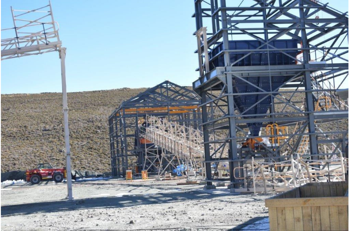
Figure 15: Construction of the dense media separation (“DMS”) feed bin module (foreground) with conveyors to DMS module (background)
