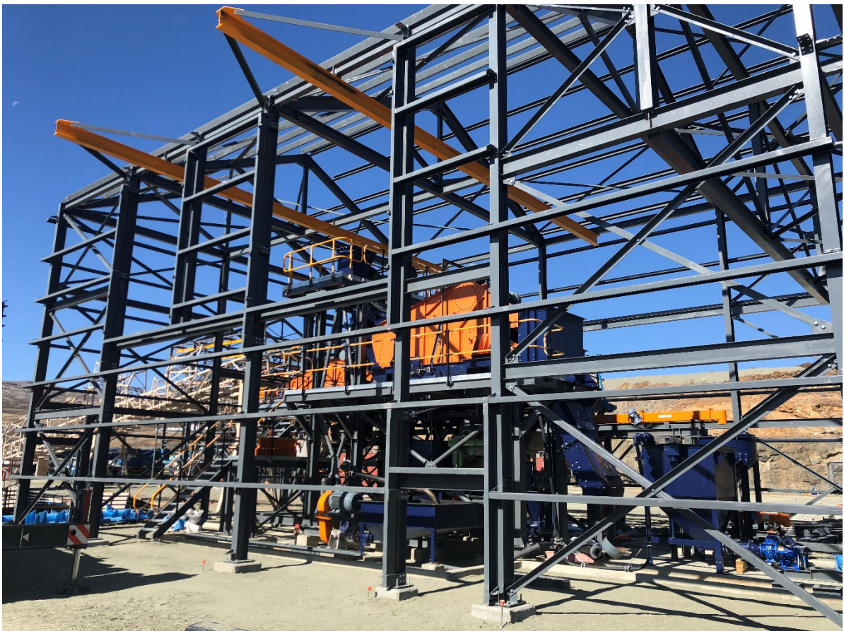
Figure 16: Construction of the DMS module
