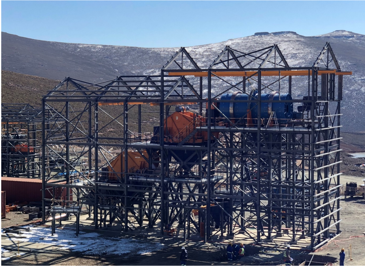
Figure 13: Construction of the scrubbing and screening module
