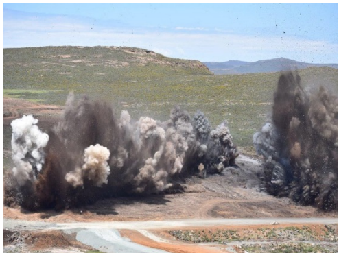
Blasting of platform for new 150 tph Mothae plant
