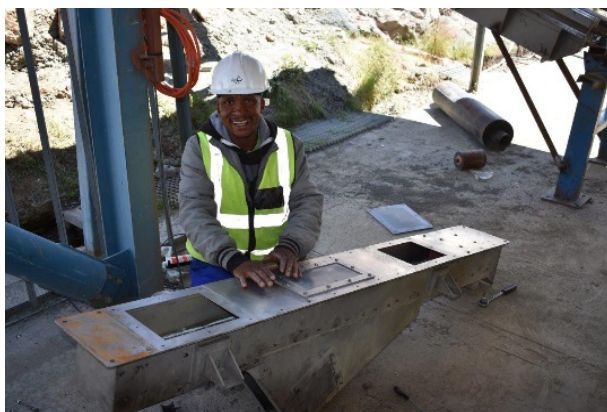
Refurbishment of a concentrate tube feeder
