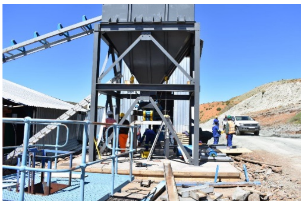
Installation of the new secondary crusher surge bin
