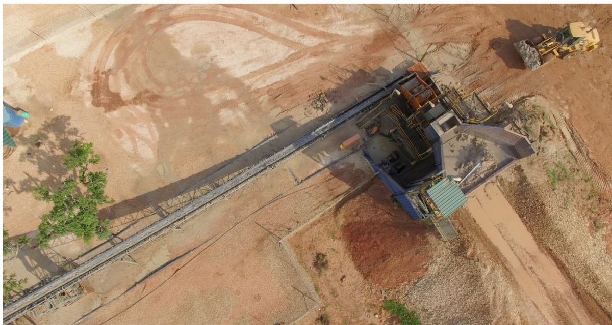
Alluvial wet front end at the Lulo production plant, Angola
