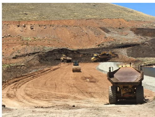
Raising the water dam wall at Mothae
