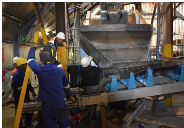
New screen discharge chute being installed
