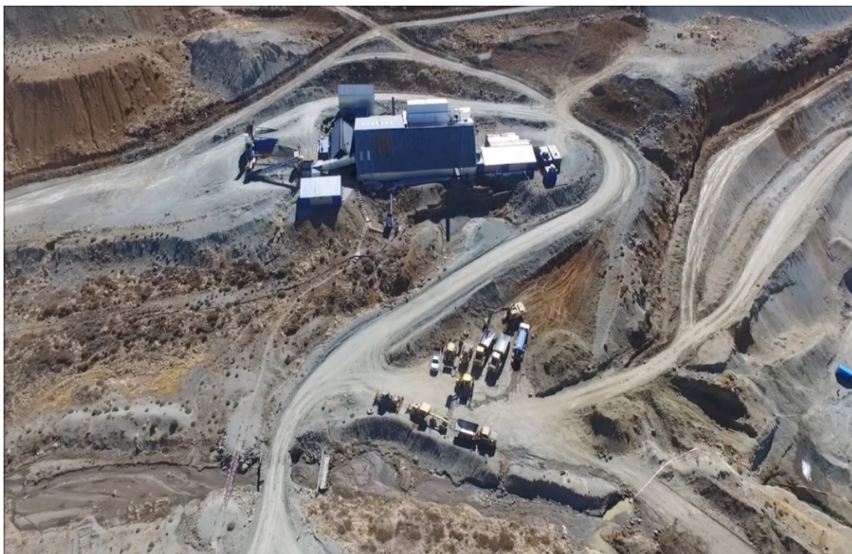
Aerial view of the existing plant infrastructure at Mothae, which is being refurbished for a preliminary bulk sampling program
