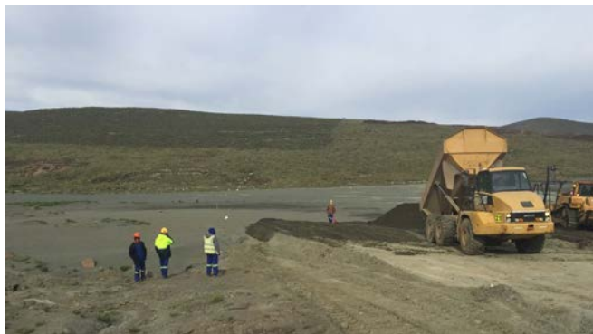
Construction of starter wall for life-of-mine slimes dam at Mothae
