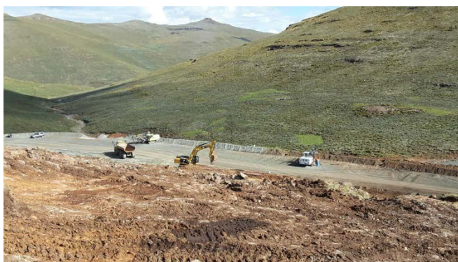
Site preparations for the new 150 tph Mothae plant
