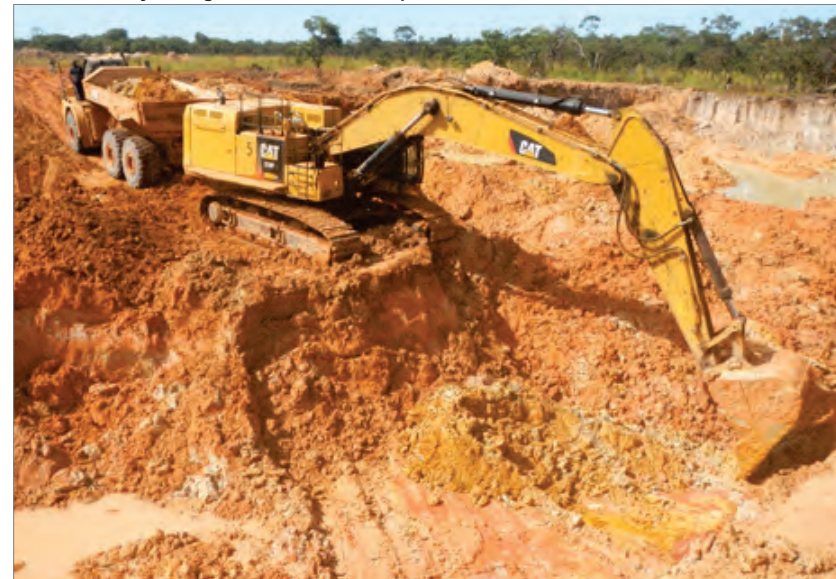
Excavation of yellow gravel at MB-28-B in April 2017
