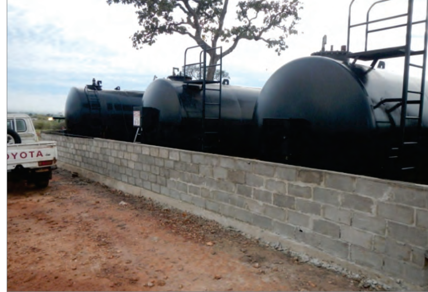
Completed bund wall around three diesel tanks
