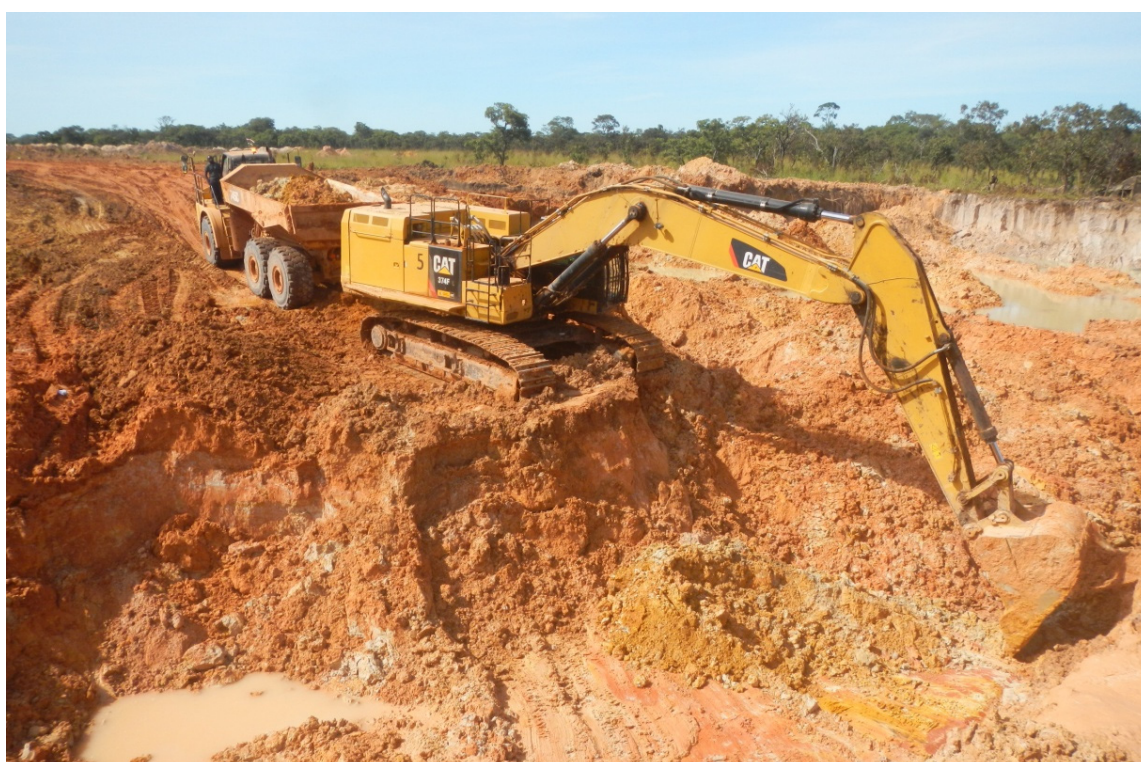
Excavation of alluvial gravels from Lulo Mining Block 8 during the Quarter
