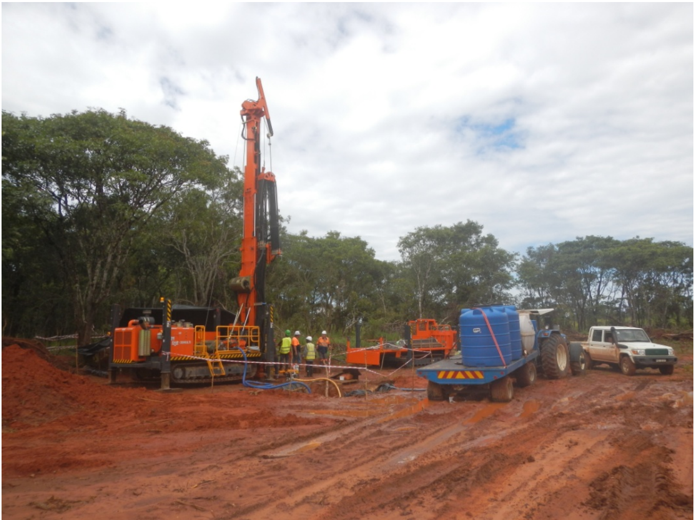
The high-capability Hanjin D&B35 drilling rig, which arrived on site during the Quarter and has since been commissioned
