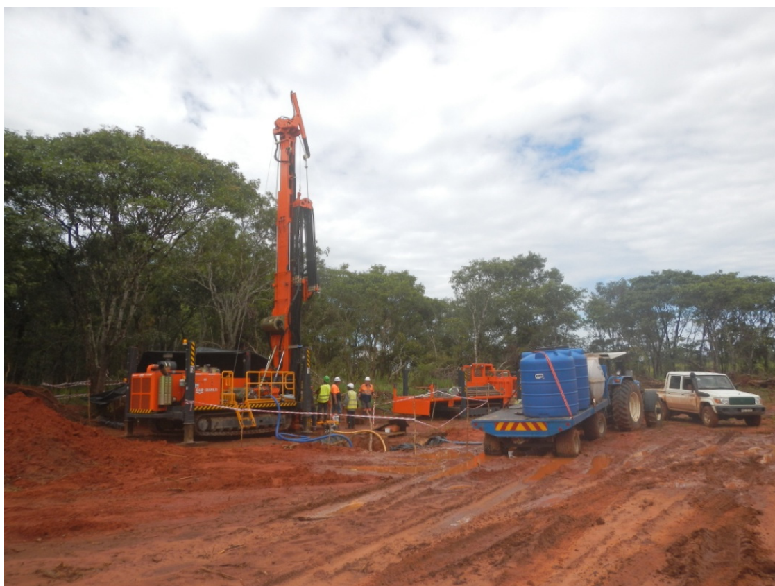
New Hanjin D&B drilling rig in operation at Lulo
