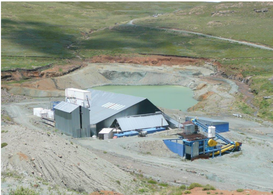
Figure 3: View showing proximity of existing plant to the South Lobe
