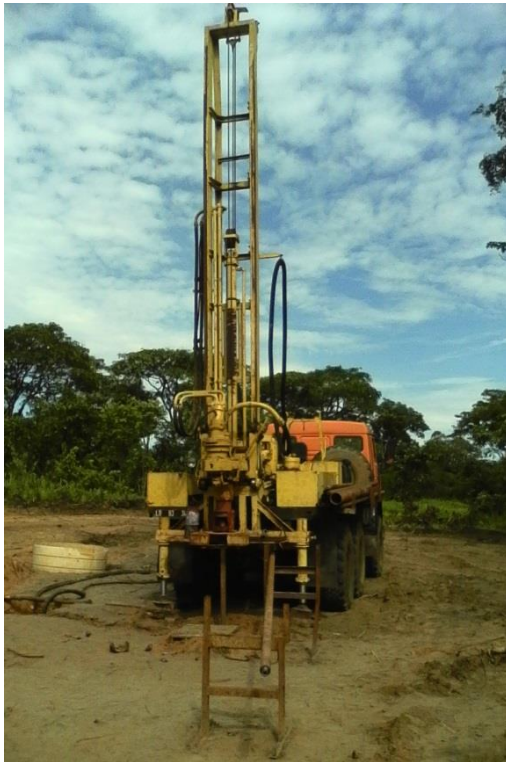
Rosanstroi contract rig drilling at Lulo
