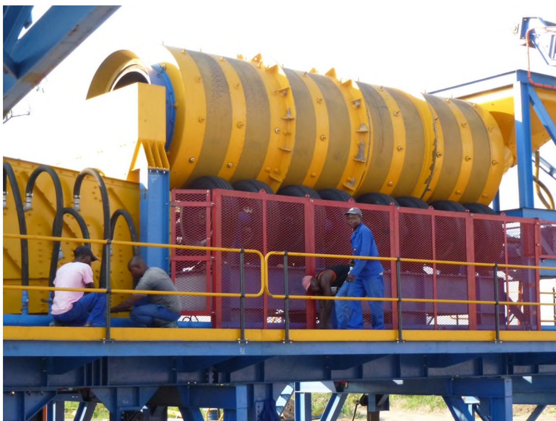
Lucapa's new 50 tonne per hour DMS diamond plant
