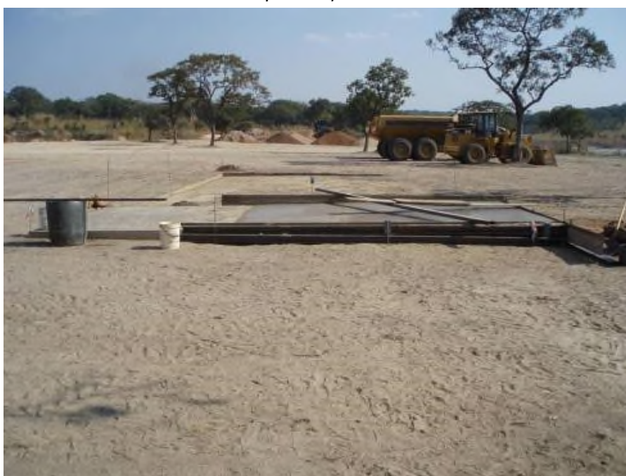
New DMS plant scrubber base being constructed
