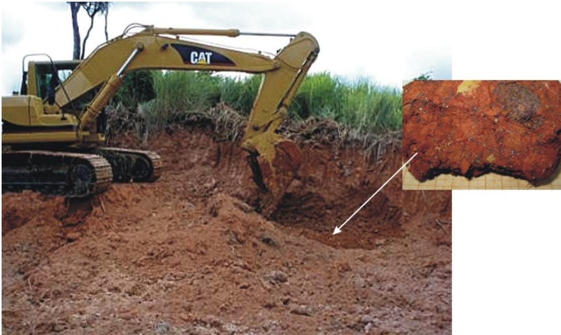
Figure 3: Bulk sample pit at Se019, showing weathered kimberlite
