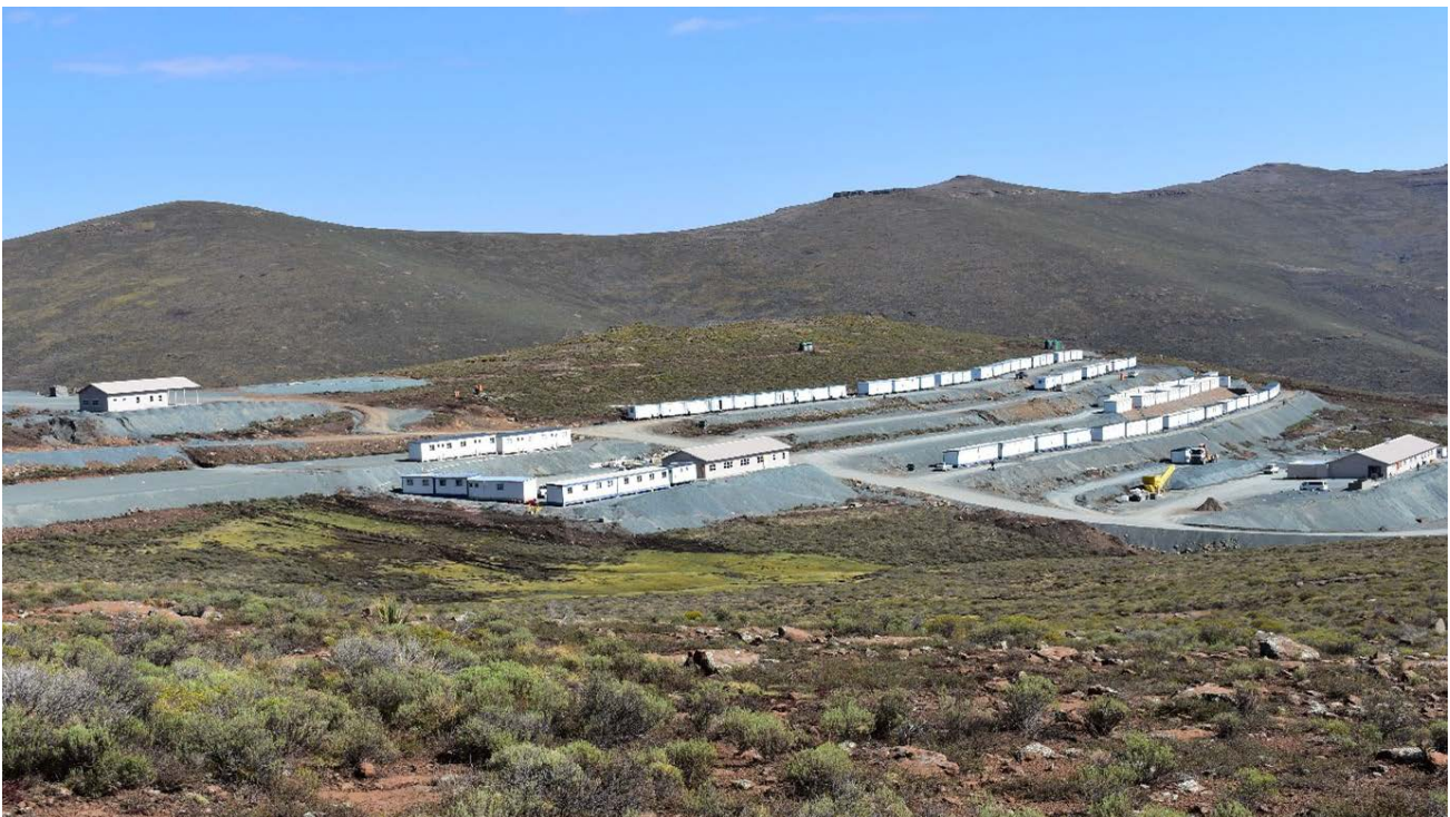
Relocation of new camp and mine offices at Mothae mine in Lesotho
