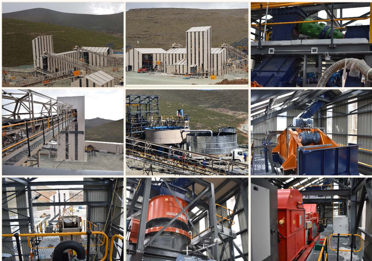
Figure 3: The 1.1Mtpa Mothae diamond plant under construction
