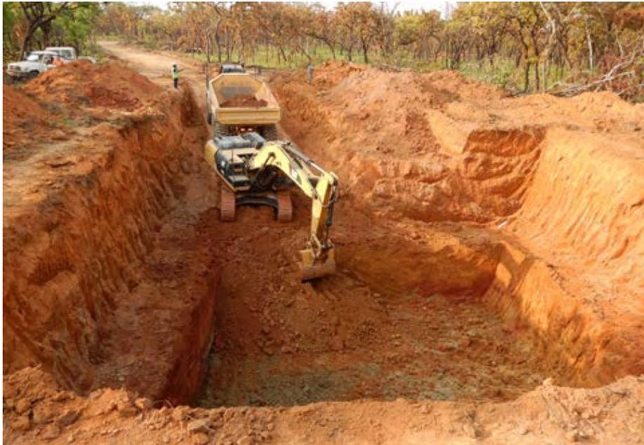
Figure 1: Kimberlite material from L104 being excavated for bulk sampling
