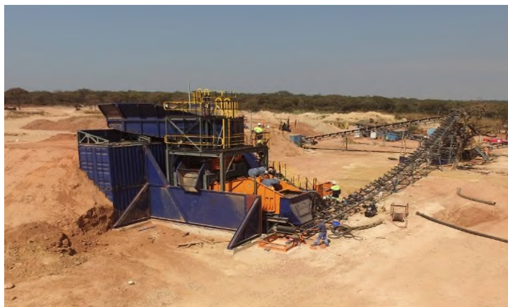
The new wet front end module at Lulo
